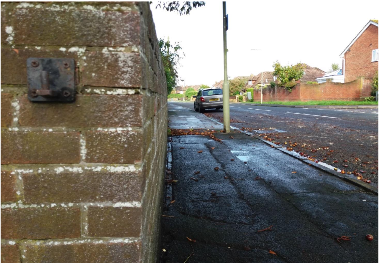
View adjacent to wall looking west
