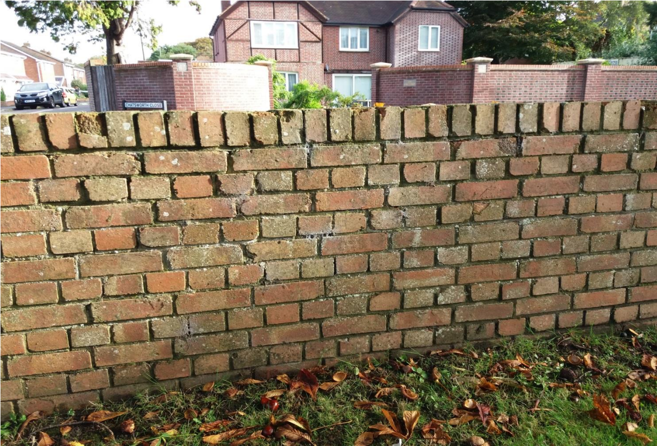
Appendix D – front garden wall.
